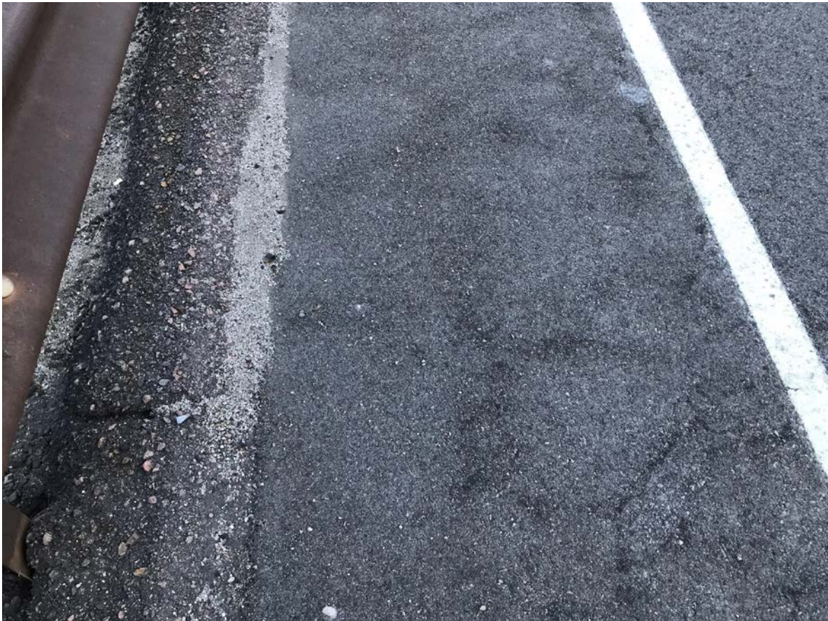
Figure 20. Slight Raveling in Control Section at Approximately MM262.05
