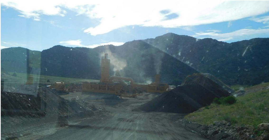
Figure 2. Overview of Asphalt Plant Site
