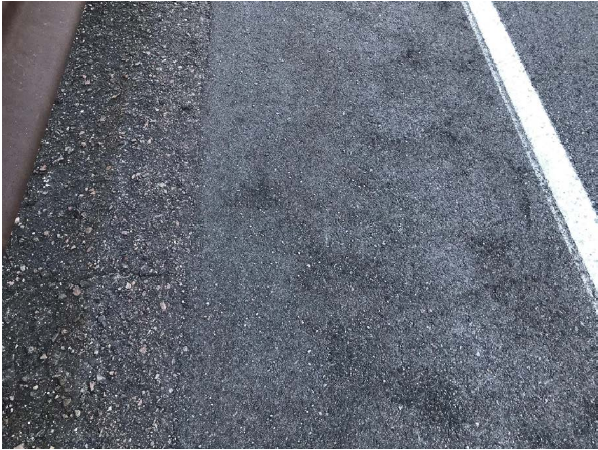
Figure 20. Slight Raveling in Control Section at Approximately MM262.05
